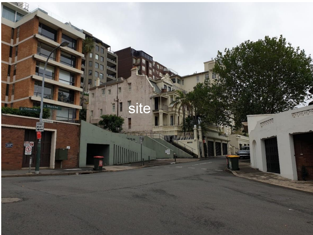
Figure 3: The subject site and surrounding development viewed from Billyard Avenue, looking north-west
