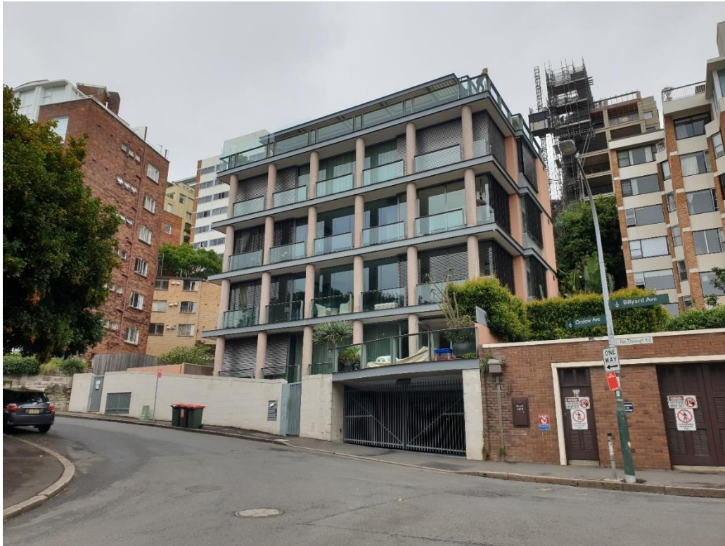
Figure 13: Residential flat building at 1-3 Onslow Avenue (left) and adjacent substation at 1A Onslow Avenue (right) to the south of the subject site, looking west
