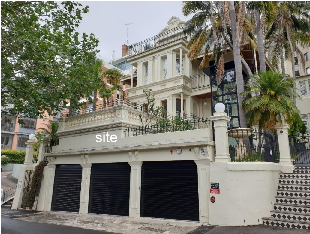
Figure 2: The subject site viewed from Billyard Avenue, looking south-west
